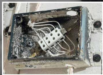
Metal enclosures and ceramic terminals remain in good condition.
